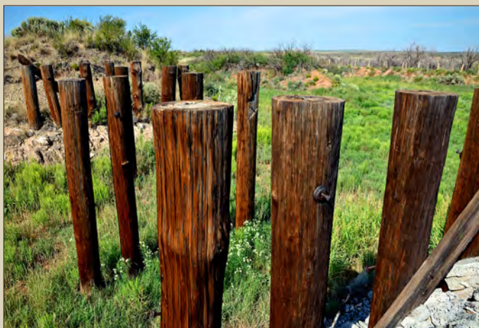
Wooden pilings, installed not long after 1900, now stand as Stonehenge-type monuments to a way of life and travel long-vanquished. Trains were the easy and classy way to travel back when Rt 66 (in the distance) was still a primitive dusty road in many places.
