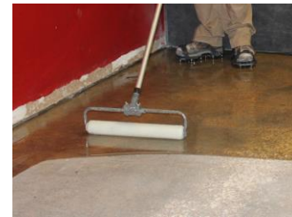
Backroll to even the coating & coverage
