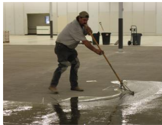
Squeegee out to proper spread rate
