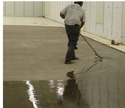
Squeegee out to proper spread
