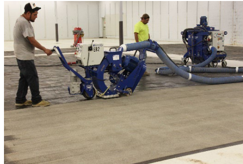
Follow by shot blasting to profile the cleaned concrete.
