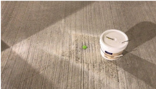
The two photos above are from a new parking deck project where the installer was faced with coating a CSP 10+ broom finish. The concrete company that finished the surface, according to specifications, called for a CSP 4 – 5 in this area, this was lost somewhere in the communications. Grinding was not allowed due to the location of the structure, so the high points of the broom finish had to be “buried” utilizing 3-coats of ACTECH 2170™ FC, incurring additional material costs.
