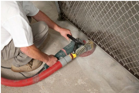
Edge-Grind; Note dust collection
