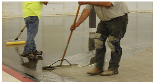
Continue on working the "wet-edge"; squeegee-backroll
