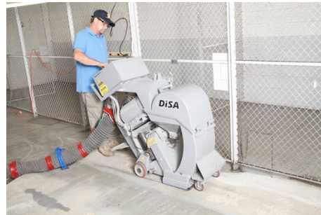
Shot Blast (or grind) up to edging
