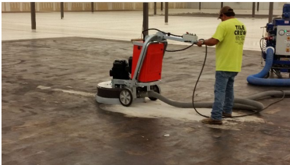
Grind to remove cutback, old adhesives, coatings and surface contaminants.
