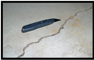
Left: Random Crack; may be static or dynamic
