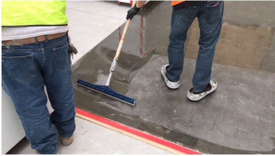
2 nd coat, pour on deck spread with a squeegee...
