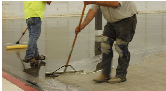
Continue on working the “wet-edge”; squeegee-backroll
