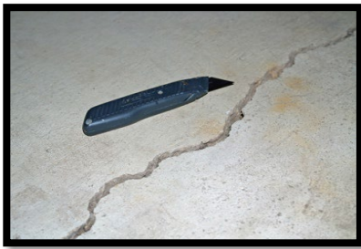
Left: Random Crack; may be static or dynamic
