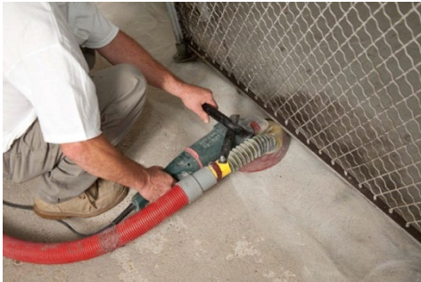
Edge-Grind; Note dust collection
