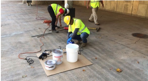
Left: A simple mix-station on cardboard
