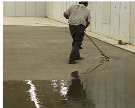
Squeegee out to proper spread rate
