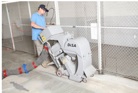
Shot Blast (or grind) up to edging
