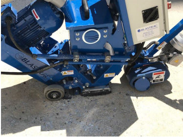
Shot blast the deck to a CSP 3-4
