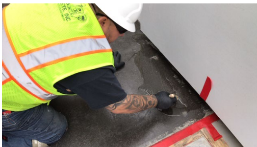
Cutting in with a brush on second coat
