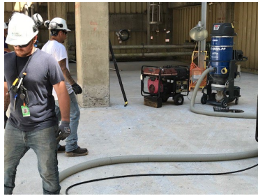
Magnet “broom” to remove shot, vacuum-clean deck prior to start.
