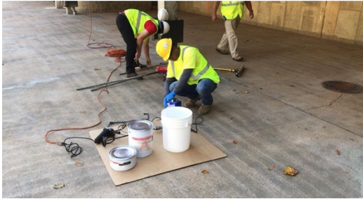
Left: A simple mix-station on cardboard
