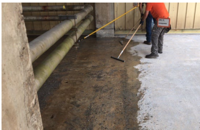
Coating under the pipes.
