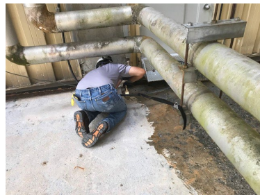
Cutting in around perimeter and under pipes and around columns.
