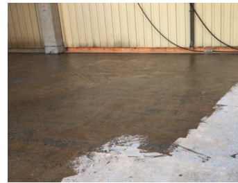
Note how the thinned material is “wetting” the concrete.
