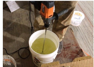
Mixing the ACTECH 2170™ FC and acetone in a 5-gallon bucket.
