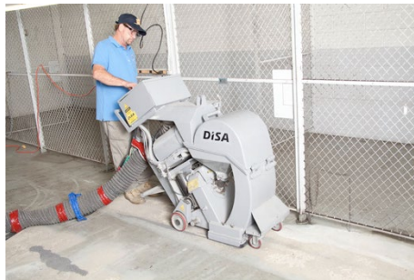
Shot Blast (or grind) up to edging
