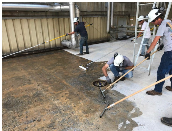
Squeegee, backrolling and cutting in around drain.
