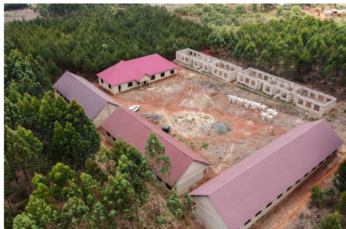
Luftansicht der Mahenge Secondary School
