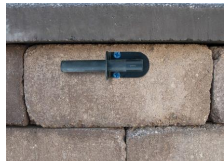
Figure 6.5 – Fasten down the bracket
