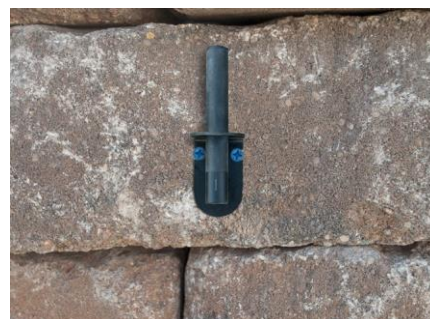
Figure 6.9 – Fasten down the bracket
