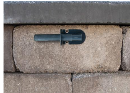
Figure 6.4 – Dry fit the bracket
