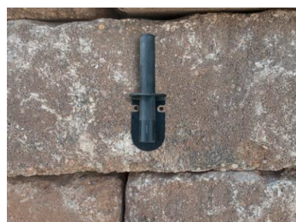
Figure 6.8 – Dry fit the bracket
