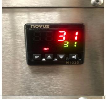
PV (Process Value) is the actual temperature of the vessel is shown in RED
