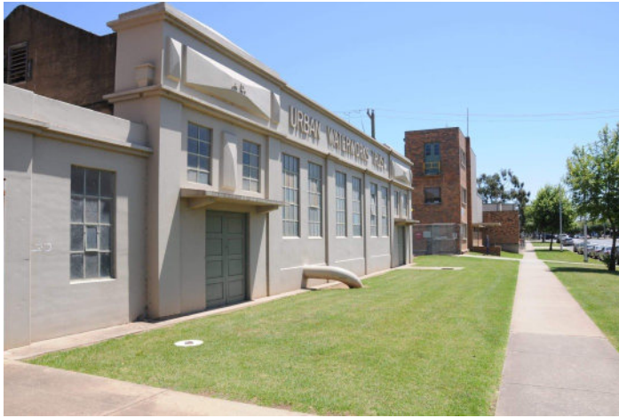
Shepparton Water Treatment Plant
