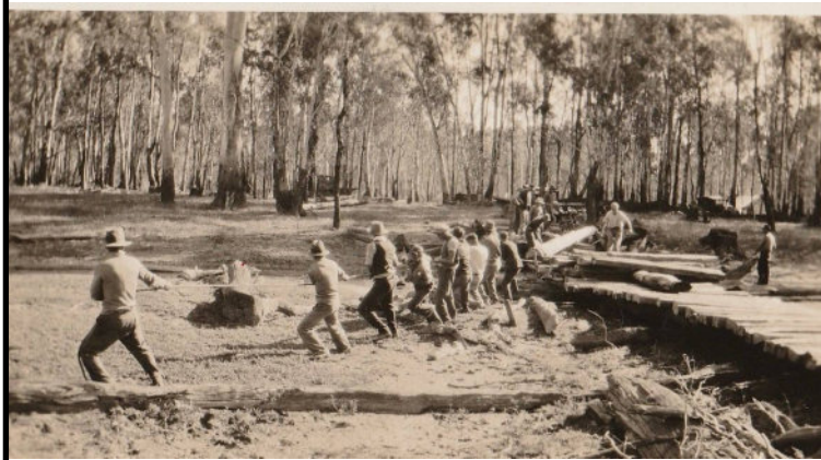
Pictured below— construction of bridge on Barmah Creek.
