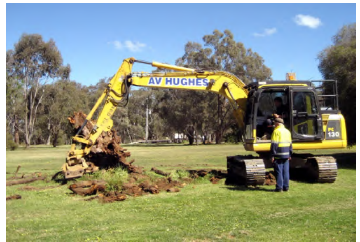
Above: Andrew Hughes doing a great job removing stumps.
