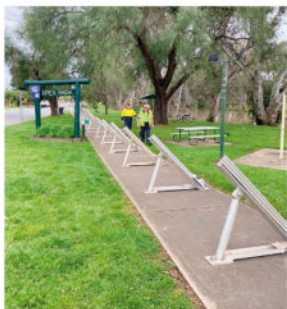
Council staff set up the Nathalia Levee.
