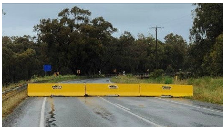
No access over McCoys Bridge due to the flooding and damage to the bridge.
