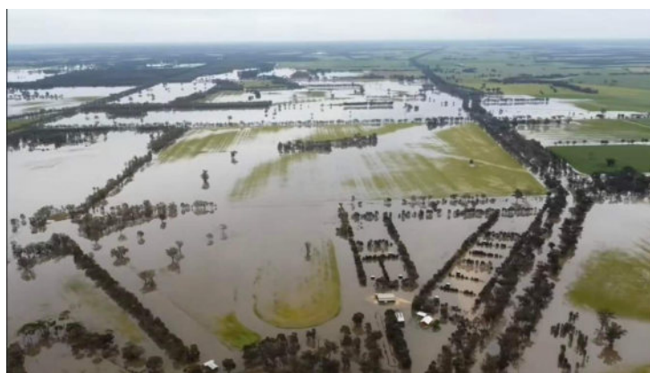
Corner of Barmah-Shepparton Rd & Murray Valley Highway, Nathalia South Recreation Reserve - trotting track, GoKart track & shooting range, all under water.
