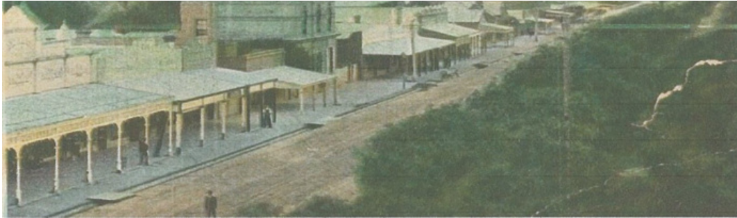
Many shops on the east side of Blake Street, Nathalia were destroyed by fire.
