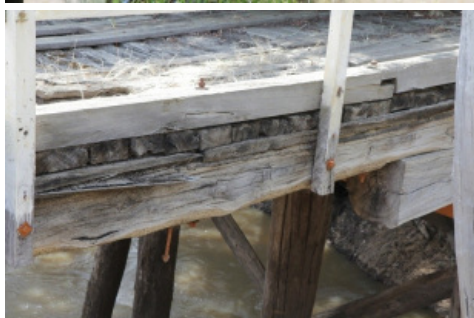
Vertical chopping axe cuts can still be seen on the red gum bridge beams.
