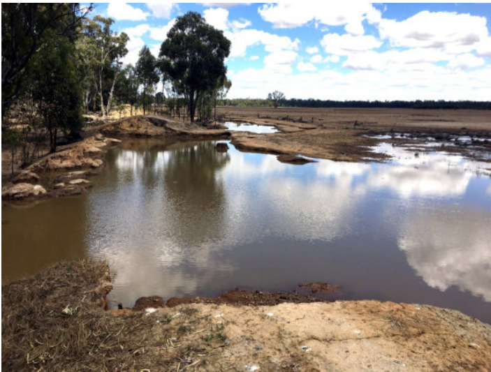
340metres of levee bank destroyed at Loch Garry.
