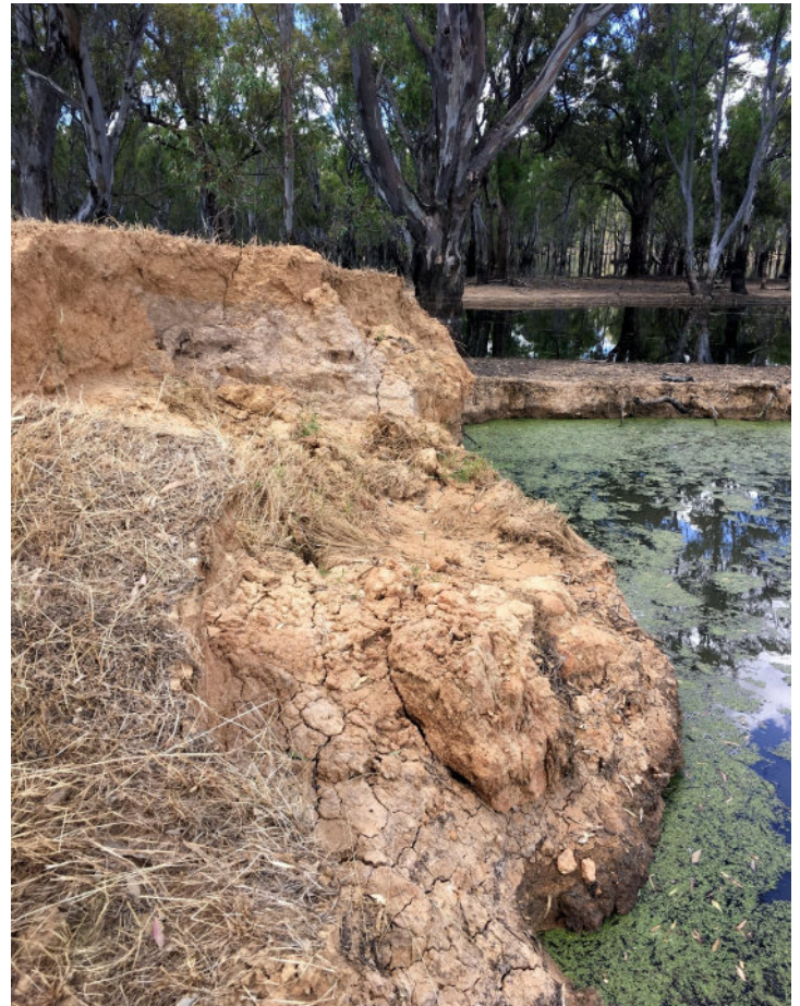
10ft hole caused by force of the flood water.
