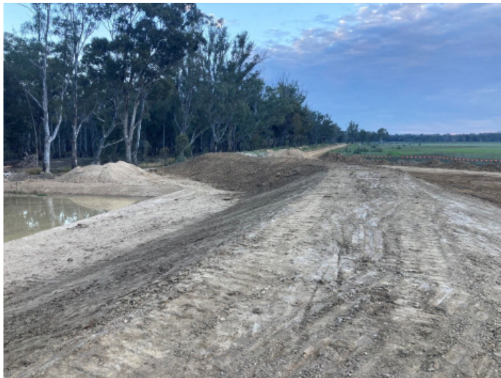
Completed Levee
