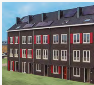
Nobelhorst. Residential building. Almere, Nederland. Aquarea.
