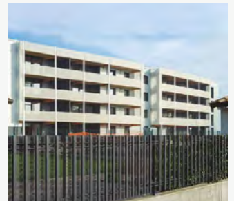
Crosslight House. Residential building. Mulazzano, Italy. PACi and nanoe™ X.
