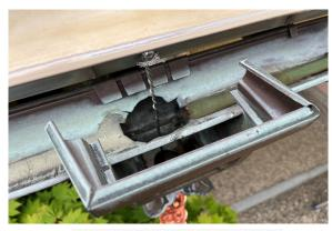
(3)-2 If the provided hook is not long enough or if additional reinforcement is necessary, please hang it from the eaves or fascia using a screw and wire.
