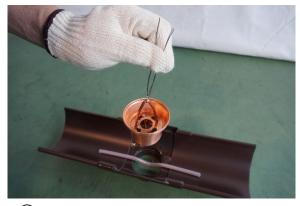
2 Attach stainless steel wire to the first chain and prepare to hang it.
