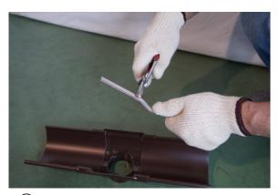
(1) Bend the hook to fit the diameter of the downspout outlet. The covering on the hook prevents electrical corrosion with the chain. Do not remove it.
