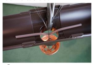
3 Hang it as close to the spout as possible to prevent the rain from splattering. It would be even better to crimp the downspout so that it tapers in.
