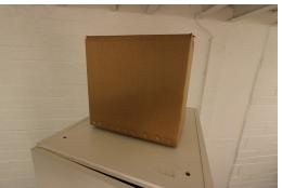
The silencer can sit on top of the vent hole and will reduce the air noise from the fan
