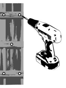
5. Set shutters aside for a moment, and use <u>1/4" bit</u> to drill into holes in the wall from the previous step. This will widen the holes in the wall sufficiently to accept wall anchors.
