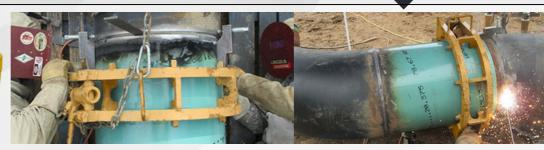
The Sawyer Mfg. Ratchet Cage Clamp provides extra strength to align large diameter pipe. Quality steel construction for consistent and accurate pipe-to-pipe fit-up. Fast, simple, strong; the Ratchet Clamp gets the job done.
