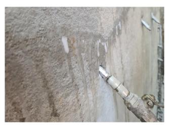
TamPur 150 ECO is a single component hydrophilic polyurethane in combination with polyether polyols. It only reacts when it comes in contact with water to form a flexible polyurethane seal.
