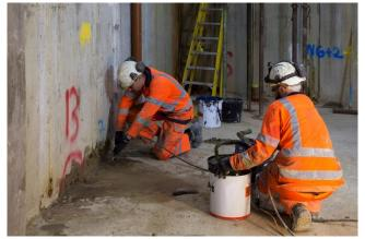
TamPur 130 is part of our new ECO range and is a single component, high foaming, semi flexible water reactive polyurethane injection resin. TamPur 130 (ECO Range) has been formulated to effectively seal cracks and joints in construction that exhibit a degree of movement, forming a semi flexible, closed cell foam sealant. The reaction speed of the resin can be adjusted using TamKat 130 providing flexibility on the job site. TamPur 130 (ECO Range) is phthalate free and environmentally friendly.
