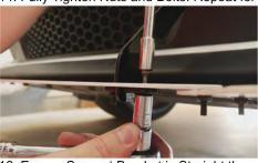
16. Ensure Support Bracket is Straight then Attach to Underside of Bumper with 2 Pointed Screws and Silver Lock Washers. Press Up Hard on Screw to Penetrate Plastic and Get it Started then Fully Tighten.
