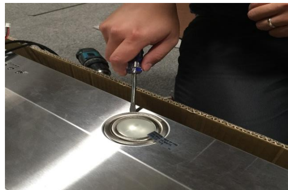
Figure 13b: Alternate Lamp Removal
