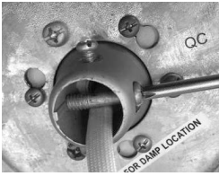
remove stopper screw and loosen set screw
