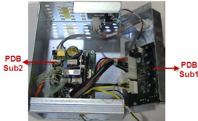
Figure 8-66 Removing Power Distribution Board
