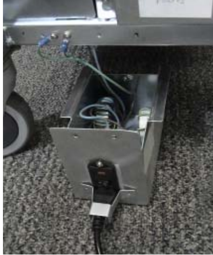
Figure 8-87 Removing Transformer Assembly
