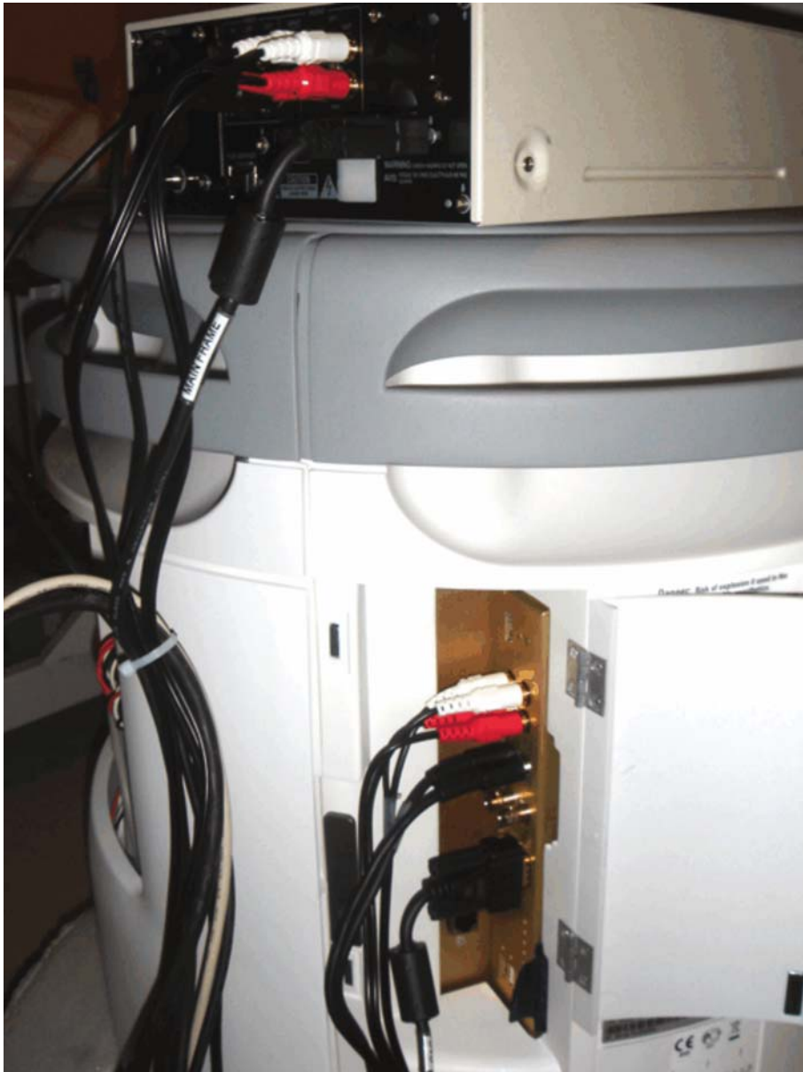
Fig. 35: DVR connected to S2000 I/O ports
