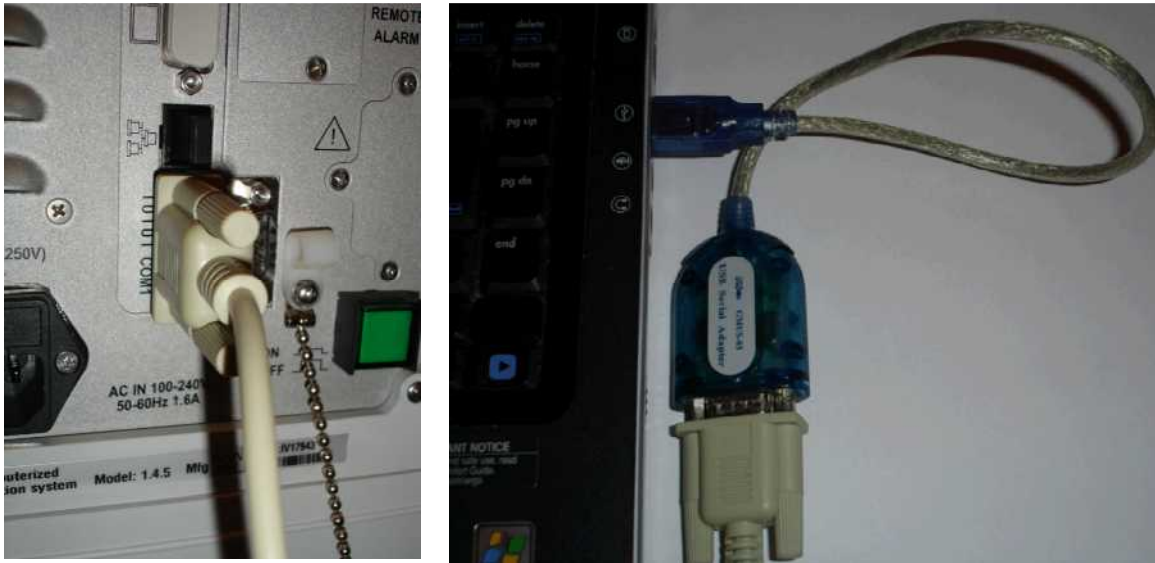
Figure 10-1 Software utilities cabling setup
