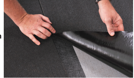
Floor Installation butt-joint membrane seams
