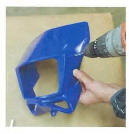
3) Drill 4 holes in the locations marked in the previous step. Use a ¼ inch drill bit. (Not provided)
