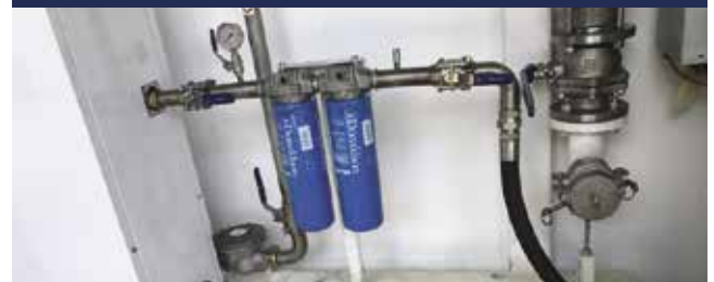
Replacement of all Particulate & Water Filters
