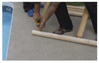
Make sure the roof supports are straight and secure each joint with a 2 ½" (64mm) screw.
