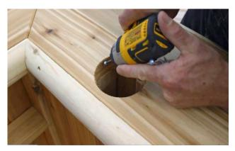
Screw the bar top to the side walls using a 2 ½" (64mm) screw by screwing on an angle through the post holes into the wall.
