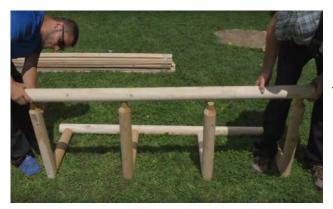
Insert the other log roof bottom side plate onto the other ends of the roof supports.
