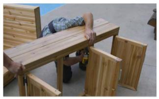
Ensure the top shelf is flush to the edge of the top of the cabinet and secure from underneath up into the top shelf with  $2 \frac{1}{2}$ " (64mm) screws.
