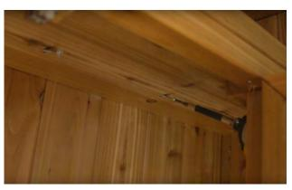
Secure the top shelf to the front wall using 2 ½" (64mm) screws in the pre-drilled holes.
