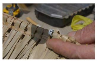
Using a hammer, fasten the palm thatch to the roof using the provided staple clips.
