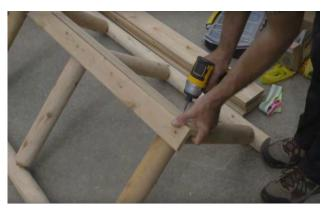
With the roof peak boards centered and overhanging on each end of the assembled roof evenly, hold them flush together at the top of the roof and secure to each roof support with a 2" (51mm) screw.
