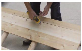
Install the roof boards (tongue & groove) working your way down each side of the roof.
