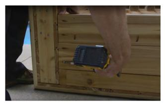
Make sure the bottom of the assembled cabinet is flush to the bottom of the tiki bar and secure with 2 ½" (64mm) screws in the pre-drilled holes.
