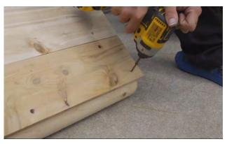
Install the roof bottom boards (straight edge on bottom) on each side.
