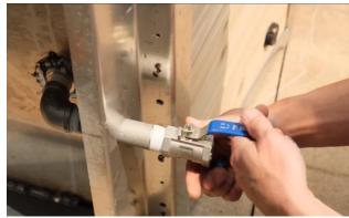
Screw the valve onto the end of the long pipe.
