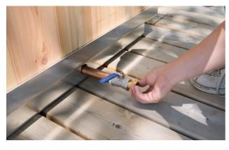
Using a pipe wrench or adjustable wrench, tighten the garden hose connector (if ordered) onto the valve.
