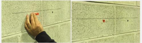
7. Place the correct frame so the holes match the plugs and fix to the wall using the stainless steel screws provided and drive provided in a drill preferably.
