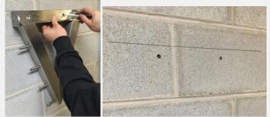
4. Repeat steps 1-3 for the other folding frame using the brickwork, roof ETC along with a tape measure to match the same height as the first folding frame.
