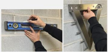
3. Hold the correct folding frame (hinged down) to the line and colour the mounting holes for drilling.
