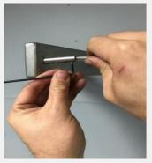
10. Hold cable as tight as possible to corresponding fitting on the opposite frame where the fitting meets the frame and cut cable approximately 5mm shorter.
