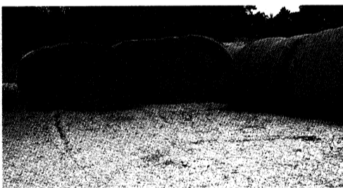
Use of a rock pad is one effective yet inexpensive way to eliminate hay/soil contact.
