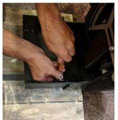
Position the Logstore legs and use the levelling feet to secure them to the body of the stove. Use a spanner or a socket wrench to fully tighten.
