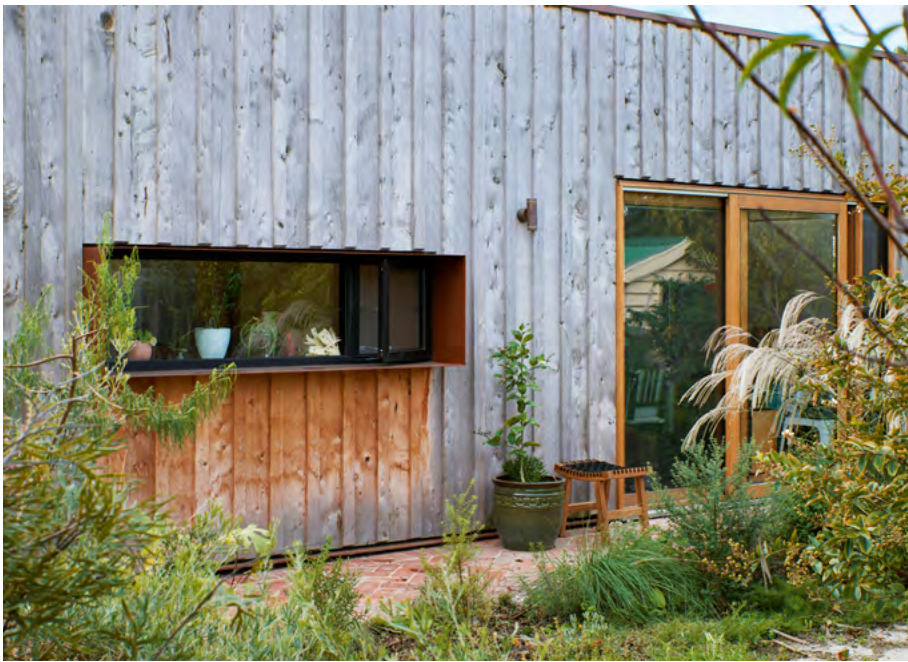
↑ Reclaimed macrocarpa boards from CERES Fair Wood were used to clad the studio. They have been left to weather to a silver-grey.
