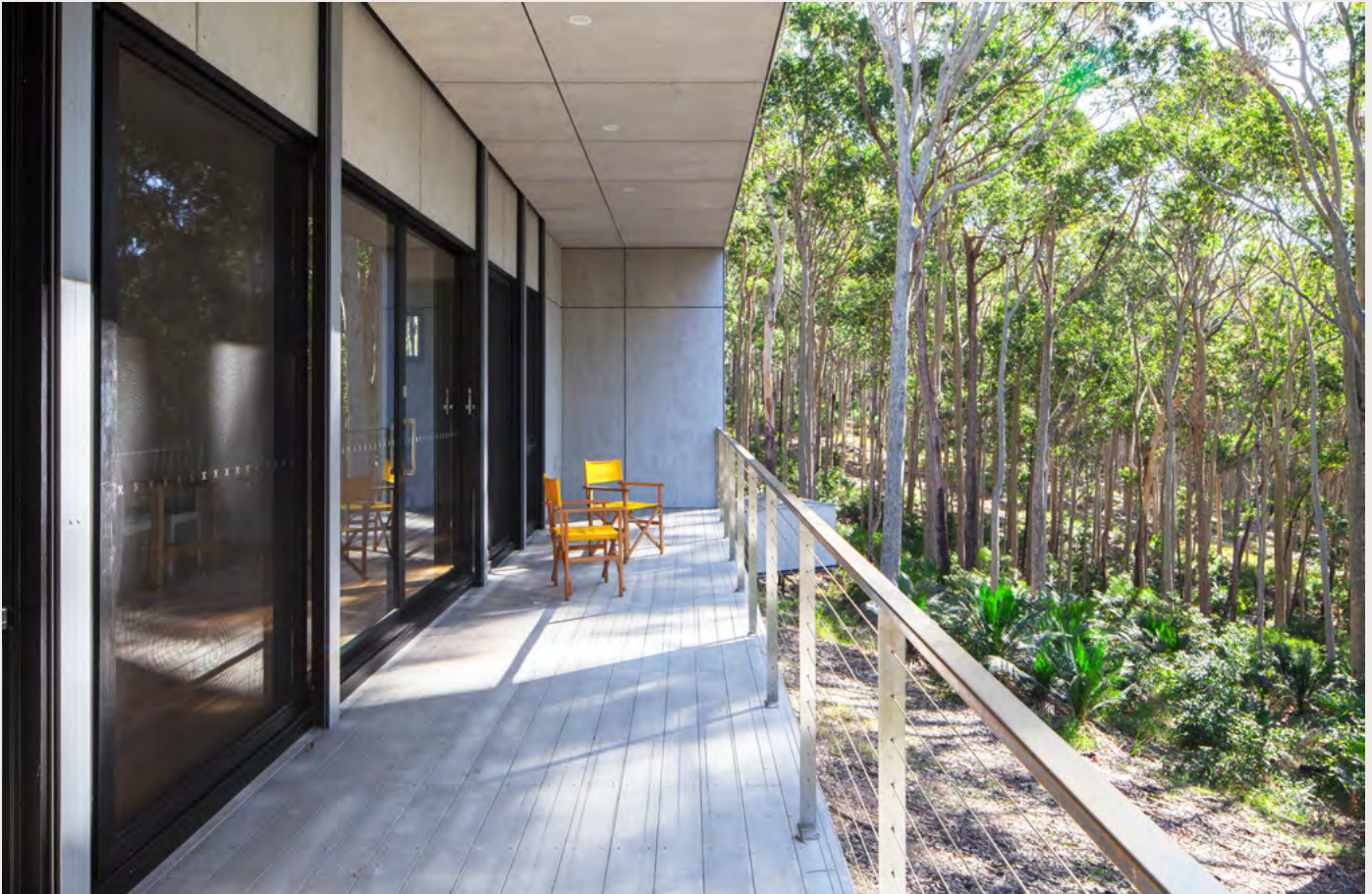
↑ Architect Thomas Caddaye opted for Ubiq Inex fibre cement boards for the deck at this house on a highly bushfire-prone site in Rosedale, NSW. The house survived the Black Summer bushfires that tore through the area in January 2020; read the full story in Sanctuary 51. Image: Ross Caddaye
