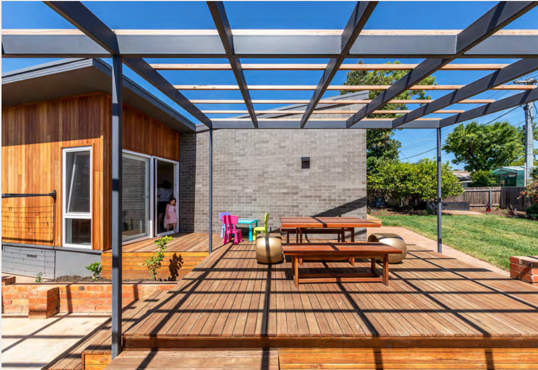
← Light House Architecture & Science specified FSC-certified Australian blackbutt ( Eucalyptus pilularis ) for the decking at this renovation and extension project in Curtin, ACT. Image: Ben Wrigley
