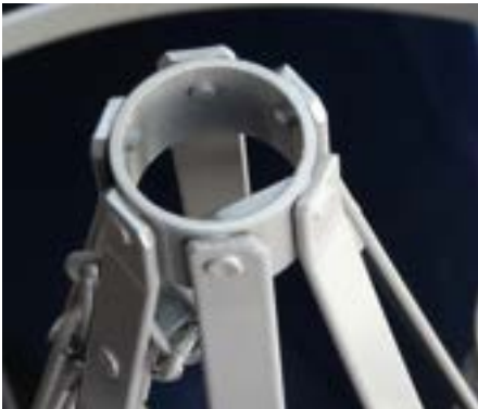
Collar with riveted end fixing.
