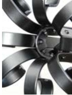
Collar with nut and bolt fixing.
