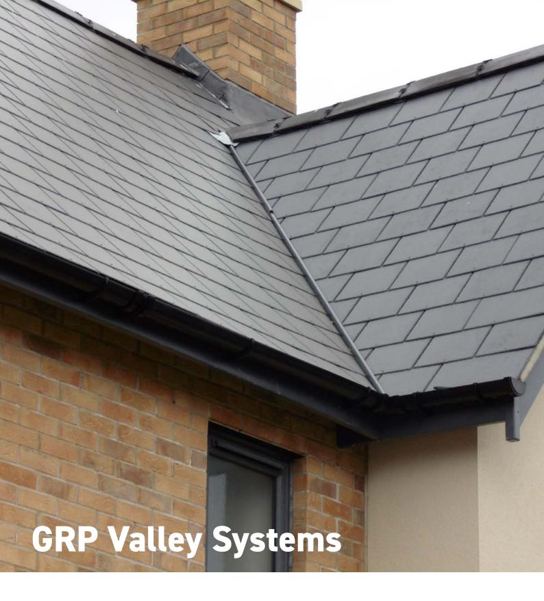
The GRP valley systems provide a range of durable and cost-effective alternatives to lead products. They are easy to install and with an array of products there is a great solution to most roof profiles.
