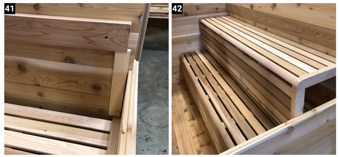
Place the bench support 2x4 on top of the bench spacer and screw Place in top bench against the back wall. to the back wall with five 2" screws.
