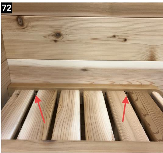
Secure porch bench to front wall using 2" screws into the pilot holes between the slats
