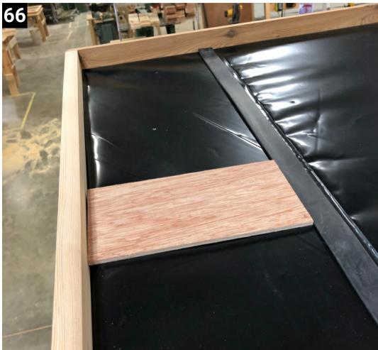
Staple or secure the neoprene strips to the roof, use the plywood spacer to properly space it from the side
