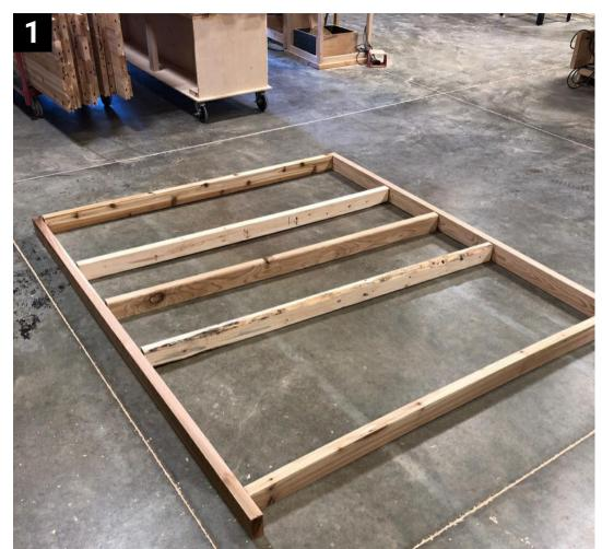
Start the assembly on a nice firm level surface. Start the floor by laying out the two 82 3/4" 2x4s and the five 67" 2x4s.
