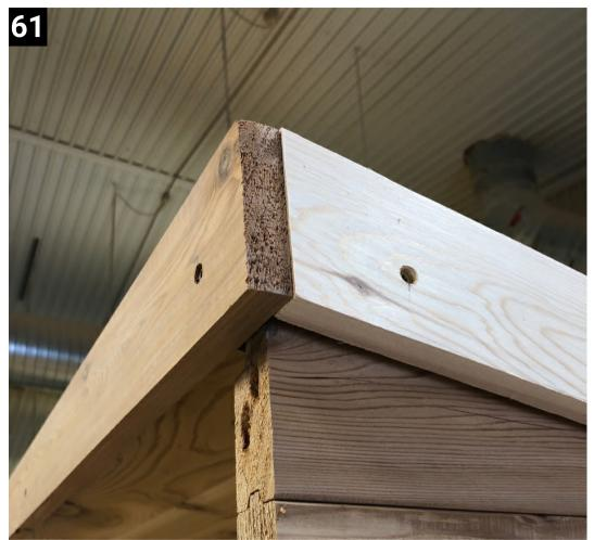
Install side pieces with the 10° mitre on them flush to the front barge board.
