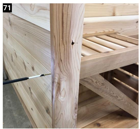
Secure the porch bench through the wall with a 3" screw into the bench arm.
