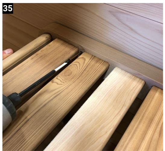
Attach the bench to the wall using 2" screws into the pilot holes between the bench slats
