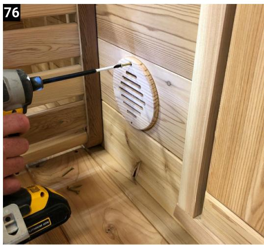
Put vents into the outside holes. Use 1 1/4" screws
