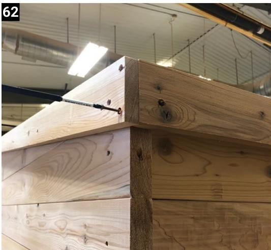
Install back barge board between the two side barge boards
