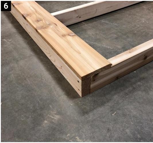
Using a tape measure, measure from corner to corner of your floor frame to make sure it's square. Measure diagonally each way and make sure the measurement is the same. If it is not the same bump the frame till it is square.
