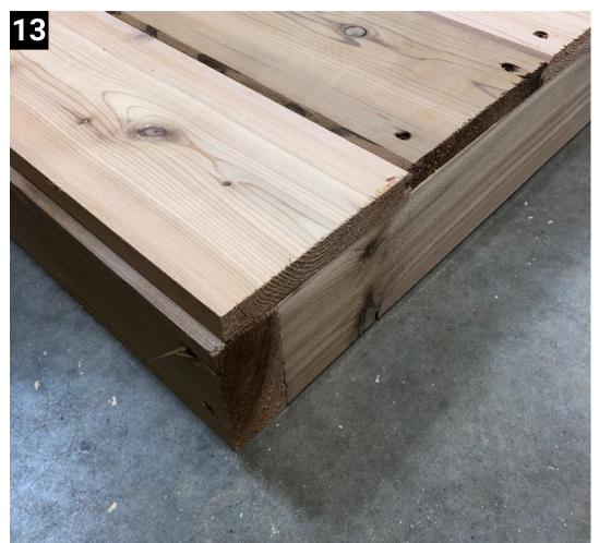
Use the other piece with a flat edge as the last board of the floor. Attach the same way as the rest
