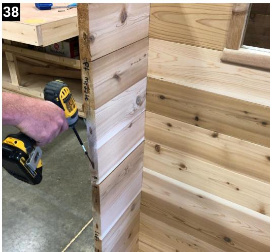
Slot in the middle of each side wall and attach to the bottom with  $4^{\prime\prime}$  screws
