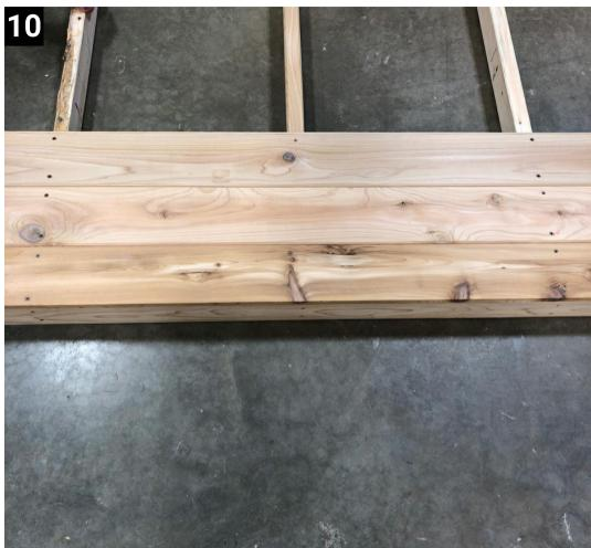
Avoid putting screws in the center 2x4 to ensure less screws under foot.
