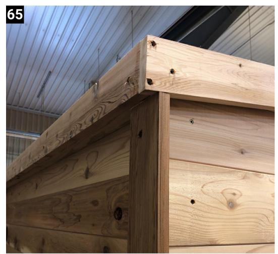
For the back barge boards, line up flush with the side barge boards.
