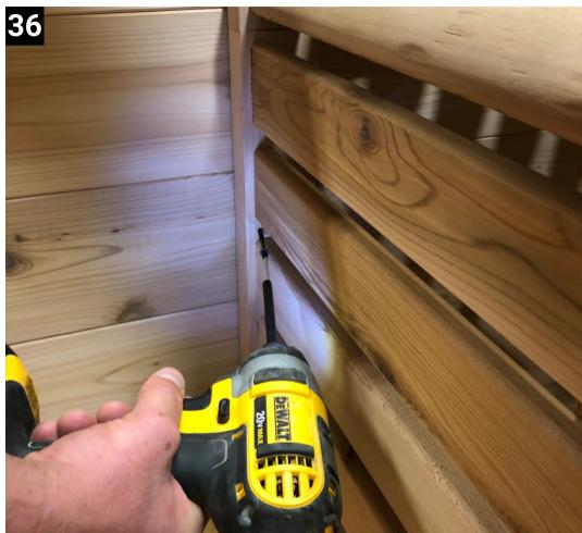
Screw the leg into the wall with 2" screws
