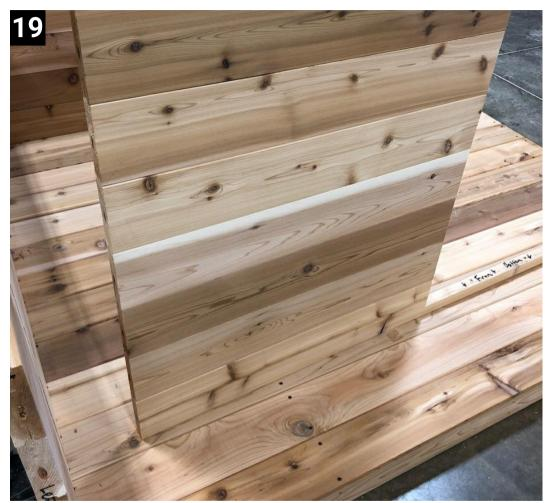
Attach one side of the front wall to the bottom piece of the front wall.
