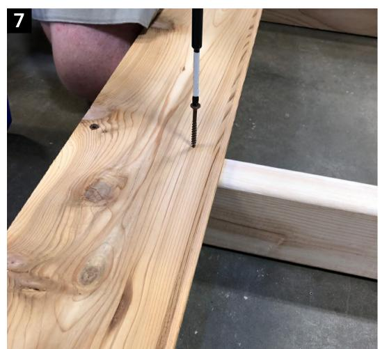
Sink two 1 3/4" screws into each 2x4 except for the center 2x4, leave it with no screws. No hot screws on bare feet.
