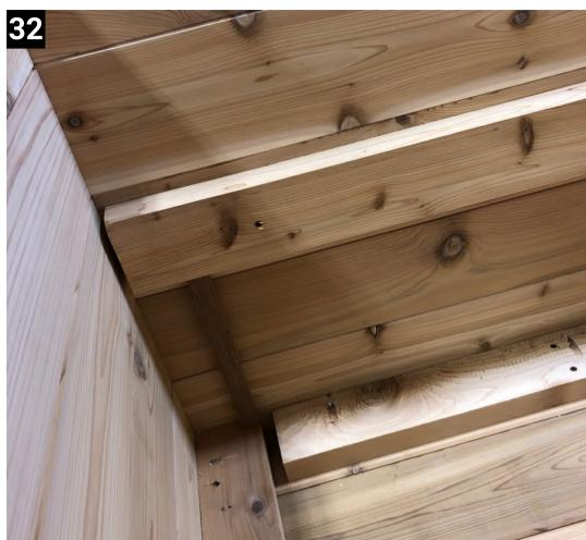
Place bench support 2x4 on top of the bench spacers and attach the 2x4 to the back wall with five 2" screws.
