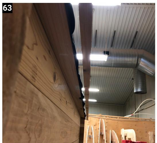
There should be a gap between the barge board and the back of the sauna
