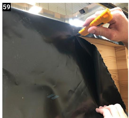
Once secured, cut roof membrane to the edge of the roof boards
