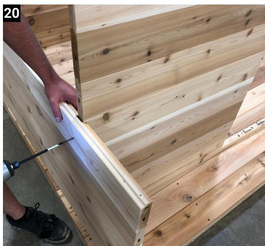
Slot the side that was just attached into the side wall. And attach using  $3^{\prime\prime}$  screws.
