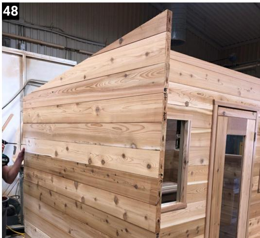
Put on both top side pieces. Screw them together with 4" screws and to the wall with 3" screws.
