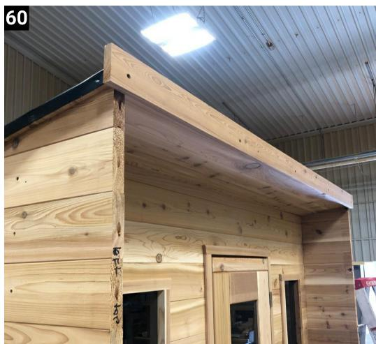
Install first 85 1/2" barge board centred on the front and 1/2" down from the inside of the roof
