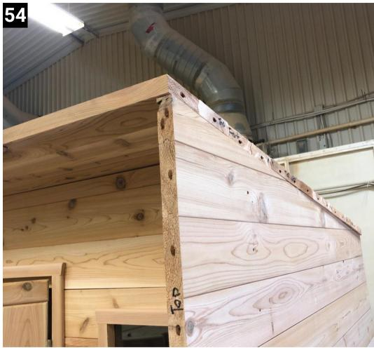
Place the top front piece on, and screw to the top middle piece with 4" screws. Make sure arrows are pointing up
