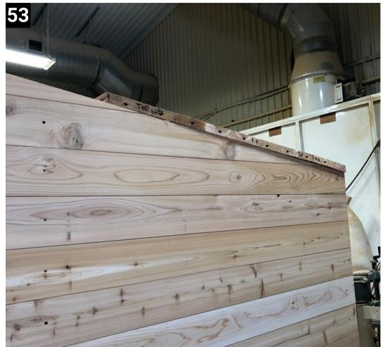
Place top middle piece on the roof and attach it to the top back piece with 4" screws
