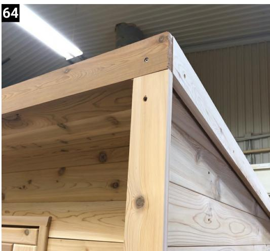
Install front barge boards flush to the edge of the top barge board, make sure it is evenly spaced all the way down
