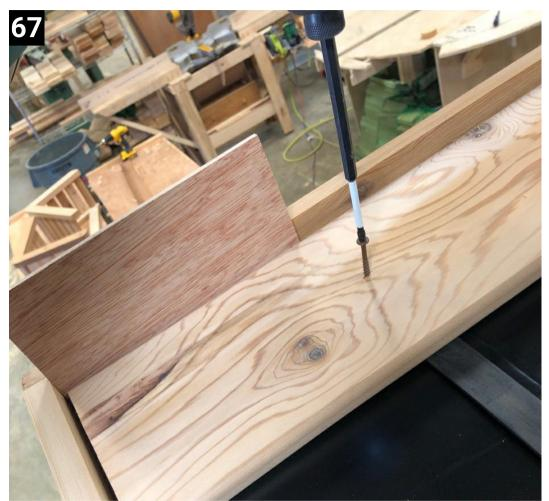
Space the first roof board with the plywood away from the front barge board. Use a 1 3/4" screw to secure it. Make sure to drive the screw through the neoprene strip
