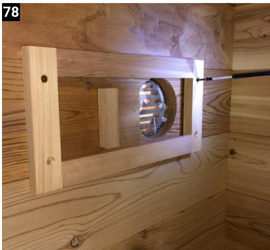
Put the vent cover over the vent holes on the inside. Make sure that they open and close fully
