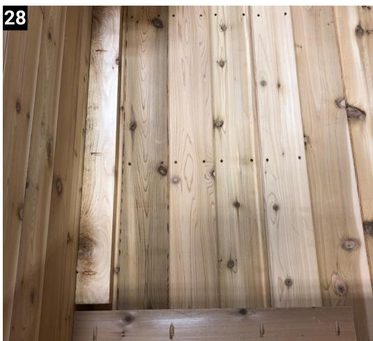
Attach the floor cleats to the floor and the walls using 3" screws down to the floor and pocket hole screws into the walls.
