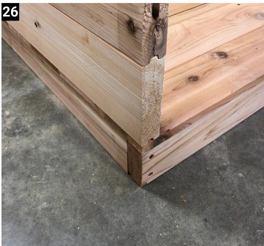
Flush up the front of the walls to the front of the floor frame, and center the sauna on the floor.
