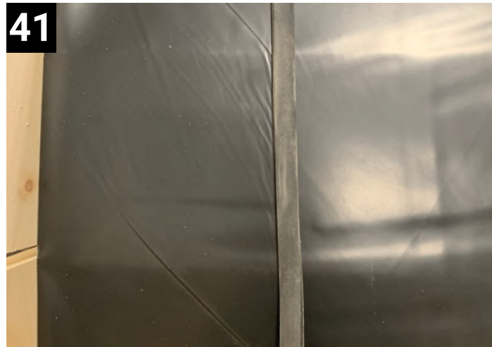
neoprene strips equal height off ground on both sides over the black plastic not onto wood. Then roof boards.
