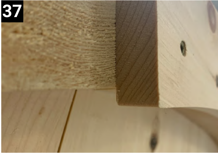
Place bottom of bargeboards 1/4" below staves.
