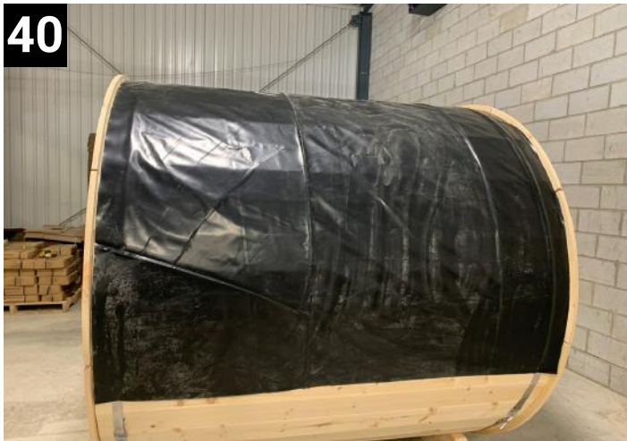
Put plastic membrane over wood staves and over each end. then neoprene strips then roof boards.
