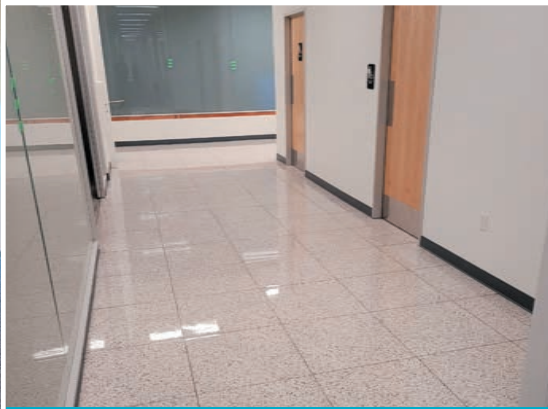
Hallway with ADA Ramp
