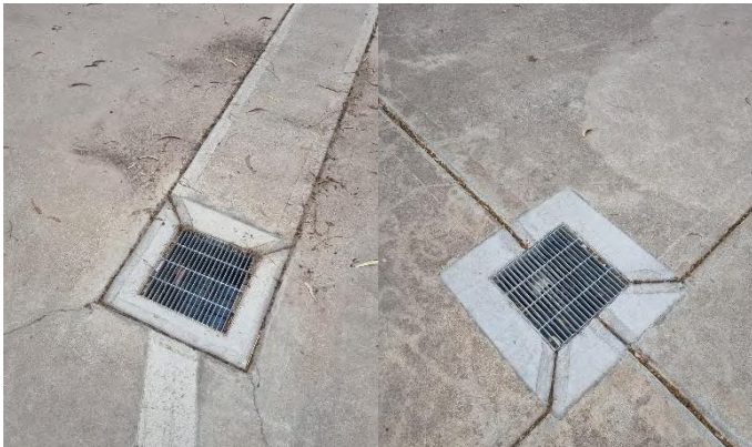
New Drains in Western Carpark
