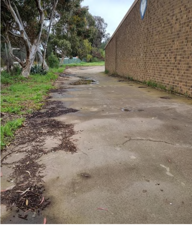
Before Carpark Sweeping
