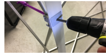
F1. Unscrew the plate and female arm from the frame hub.
