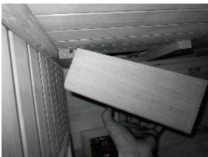
FIG 15.2 Installing the Radio Wood Housing
