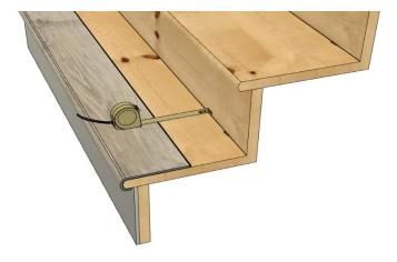
8. Transfer the measurement to a standard piece of matching flooring and cut off the excess. Be sure to cut off the groove side and leave the tongue side of the plank.
