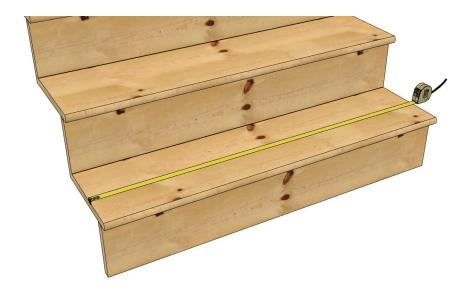
2. Transfer the measured length of the stair tread to the Luxury Vinyl Tread (LVT) nose. Best practice is to cut the tread so that the blade of the saw passes from top to bottom, this will prevent edges from fraying.
