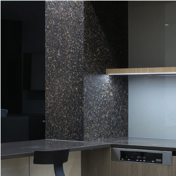
Mitre joined wall cladding with filled seam MCM Architecture for ITV Studios, London
