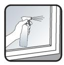
**A.** Make sure the glass is clean. Spray the film and window with solution and place the film onto the window. Slide the film and make sure it covers all edges of the window.
