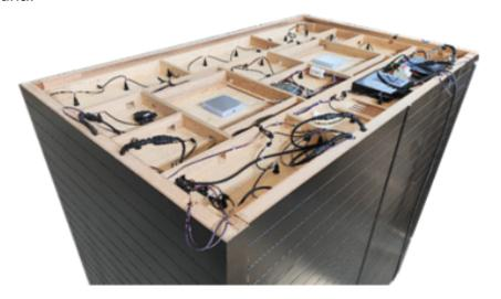
9. After the ceiling panel is in place, connect the electrical wires in the ceiling panel (male to female connectors).
