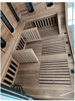
14. Take the seat panels and place them against the walls so that the LED lights in the curved edge of the bench are in the front. Push the bench flush against the walls. Open the plastic bag labeled "for support under seat." Screw two of them vertically into each end of the benches.
